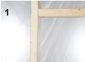
Figure 1: Determine your location for installing the Remote Device Mount. If your vertical stud is in any way bowed, twisted, unlevelled or not plumb, we recommend running a horizontal two-by-four brace between the studs to ensure that the mounting platform is 100% square, level and plumb for your Remote Device Mount. Shown in Figure 1 on the left.
