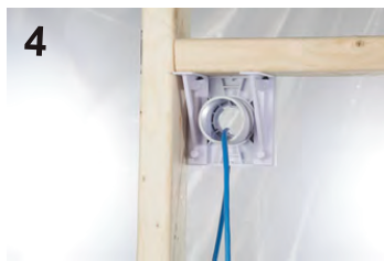
Figure 4: Mount the RDM to the two-by-four, either vertical or horizontal, using two wood screws (not included). Double check to make sure that the mount platform sticks out past the studs just under the exact depth of the drywall or wall finish. You really want the mount platform to be set back slightly from the drywall to allow room for your drywall mud or joint compound. This will make for a more flush final install. The mount legs do have a marking for 5/8 inch drywall, however we do not recommend that you solely rely on that marking for your install. You can then install the threaded insert by screwing it into the front or back of the RDM mount, turning clockwise from the front will retract the insert and turning counterclockwise will extend the insert.
