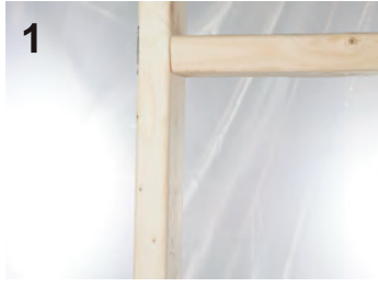
Figure 1: Determine your location for installing the Remote Device Mount. If your vertical stud is in any way bowed, twisted, unlevel or not plumb, we recommend running a horizontal two-by-four brace between the studs to ensure that the mounting platform is 100% square, level and plumb for your Remote Device Mount. Shown in Figure 1 on the left.
